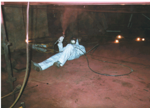
Figure 1 Industrial spray painters may have significant dermal exposure to solvents. This is due both to overspray and to the use of solvents such as white spirits as cleaning agents. Note the paint mist shown here during spray painting inside a ship's compartment. (Photo courtesy of Dr J W Cherrie, Institute of Occupational Medicine, Edinburgh).
